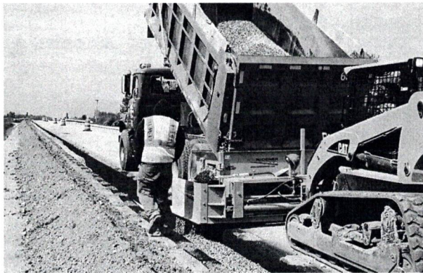
Trenching using the Road Widener.
