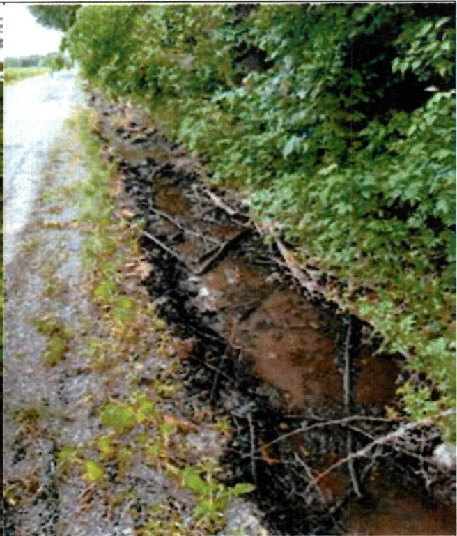
DITCH CLEANED UP
