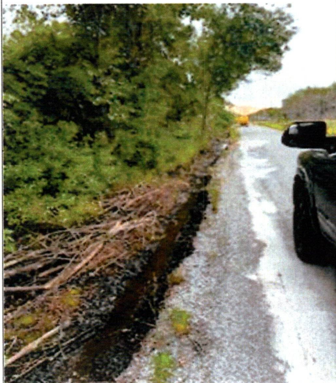
SAFE STEP ON ROADWAY
