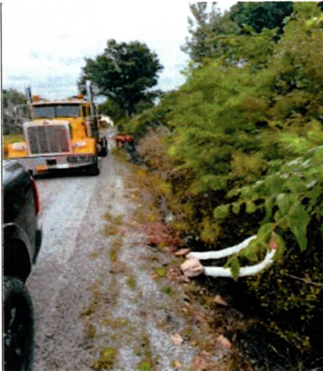
BOOMS IN DITCH & VAC TRUCK
